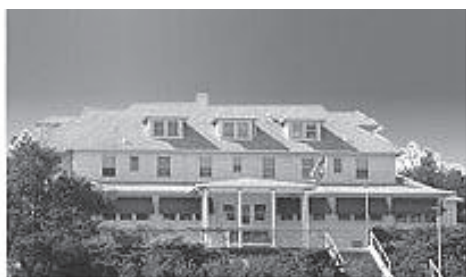
The original hospital building, built in 1928.
